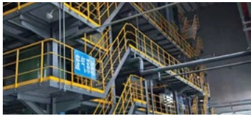
China National Building Material Equipment Group supported the launch of the world's first eco-friendly demonstration line using oil sludge to produce high-strength lightweight building aggregates
