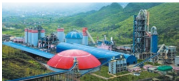
Southwest Cement has made full use of existing land resources to carry out projects involving general solid waste co-processing and alternative fuel utilization
