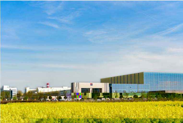
▲ The second annual 100,000-ton fiberglass production line of China Jushi's Huai'an "Zero-Carbon" Intelligent Manufacturing Base was successfully commissioned.
