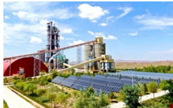
Wuzhong Saima New Type Building Materials Co., Ltd.'s "Photovoltaic + Smart Factory" project further enhanced the green and low-carbon transformation of the industrial park, adding new momentum to sustainable development.
