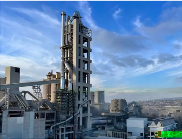
The 15MW air-cooled waste heat power generation project supporting the BASTAS Cement plant affiliated to the French VICAT Group contracted by Shanghai Triumph Energy Conservation Engineering Co., Ltd., (STEC) successfully passed the project acceptance
