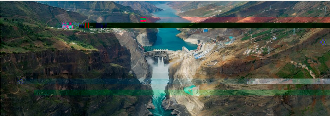
Low-heat cement is used to build the seamless dam at Baihetan Hydropower Station
